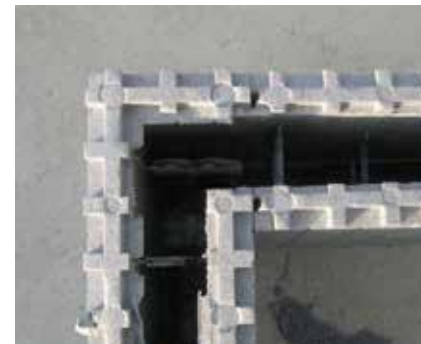
MCF 1/15 element at the corner..
