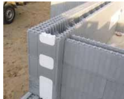
While constructing reveals and blunt wall endings, close up openings in the formwork with OH, OB and OC elements.
