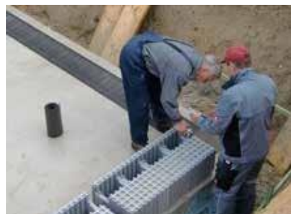
The first layer of elements.
